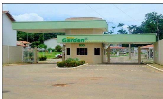
Figura 57 – Fachada do Residencial Green Garden
