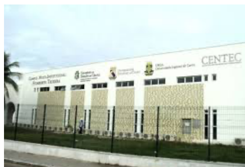
Figura 2 – Fachada principal do campus
